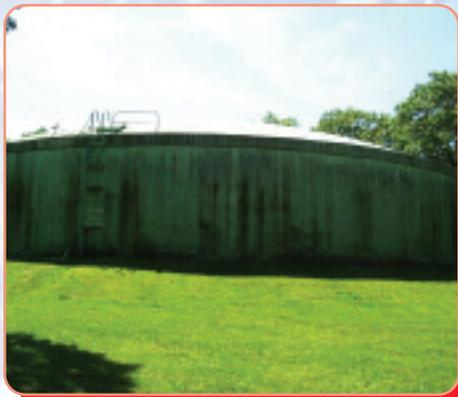
**The District is replacing the roof on its two-million-gallon ground storage tank (built in 1960) located at the Haypath Road side. What is the approximate anticipated cost?**
