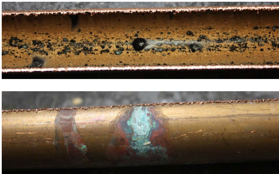
Figure A.2 – Pipe #2 interior surface (top) and exterior surface (bottom)
