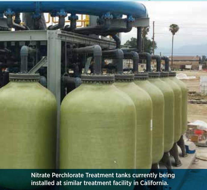
Nitrate Perchlorate Treatment tanks currently being installed at similar treatment facility in California.
