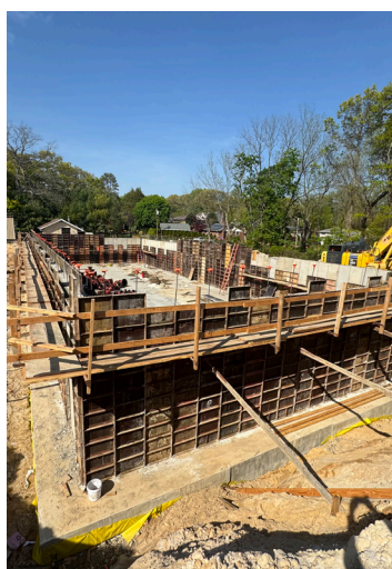
Construction at PWD's Plant 5 in May 2026.
